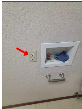
Upgrade To GFCI Outlet: Apartment Bathroom
