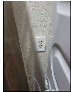
Upgrade To GFCI Outlet: Downstairs Bathroom
