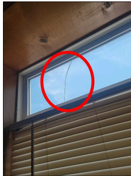
Window Glass Cracked/Broken: Upstairs Apartment Living Room
