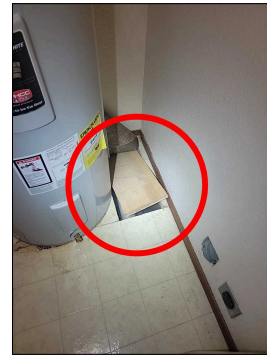
Hole In Floor Noted: Apartment Bathroom
