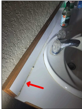
Add Caulking/Sealant: Downstairs Bathroom
